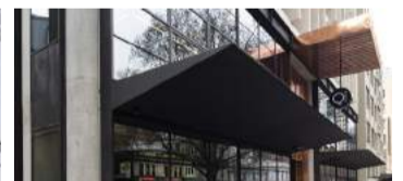
E Dark Painted Steel QT Hotel, Melbourne, Candalepas Associates
